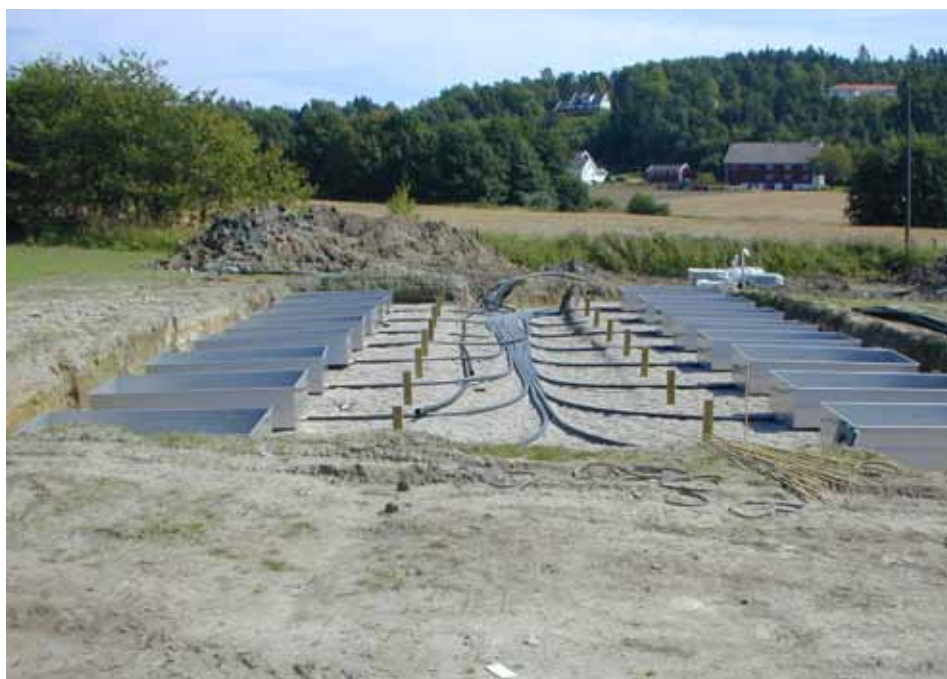
Most of STERF's studies on pesticide and nutrient leaching have been carried out in the USGA-spec. green field lysimeter facility at Bioforsk Landvik, Norway. Photo: Trygve S. Aamlid.
