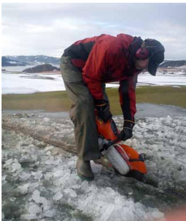
An asphalt cutter used to restore a drain out of the green.
