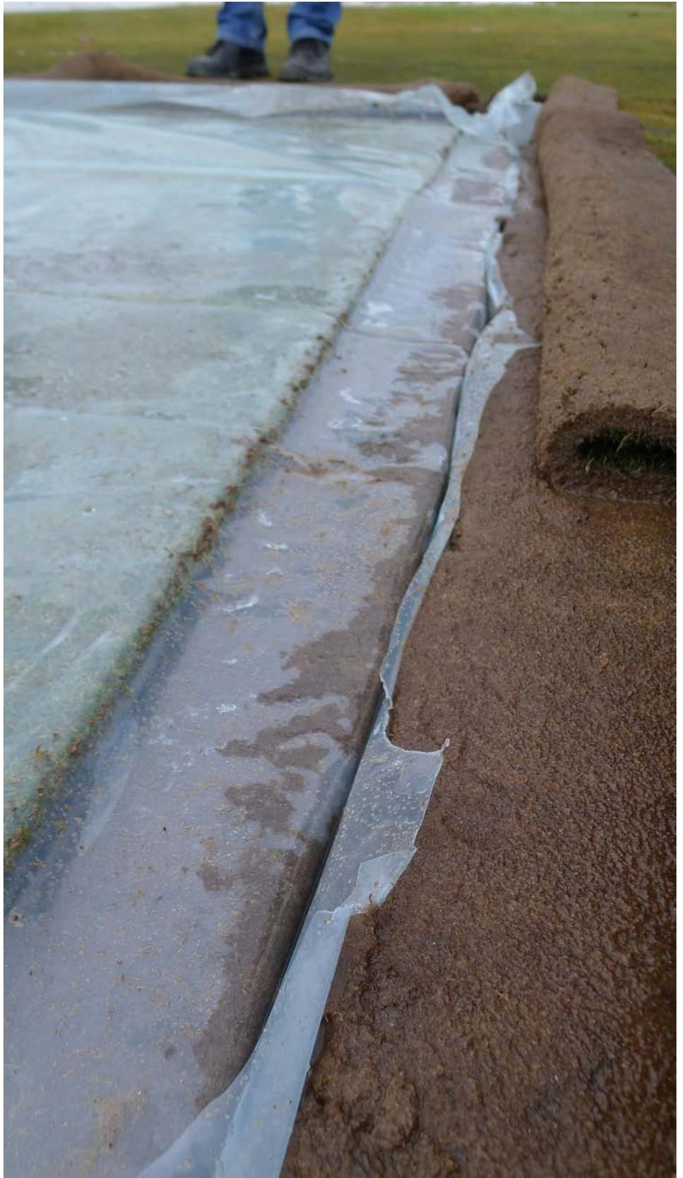
*Plastic is dug down all around the green and the edge sealed with sod from a turf cutter. This is necessary to prevent water intrusion under the covers. Photo: A. Kvalbein*
